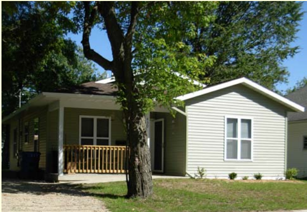
Spring 2009—Habitat for Humanity Home Walnut Street, Cadillac, Michigan Constructed by the 2008-09 CTC Building Trades Students
